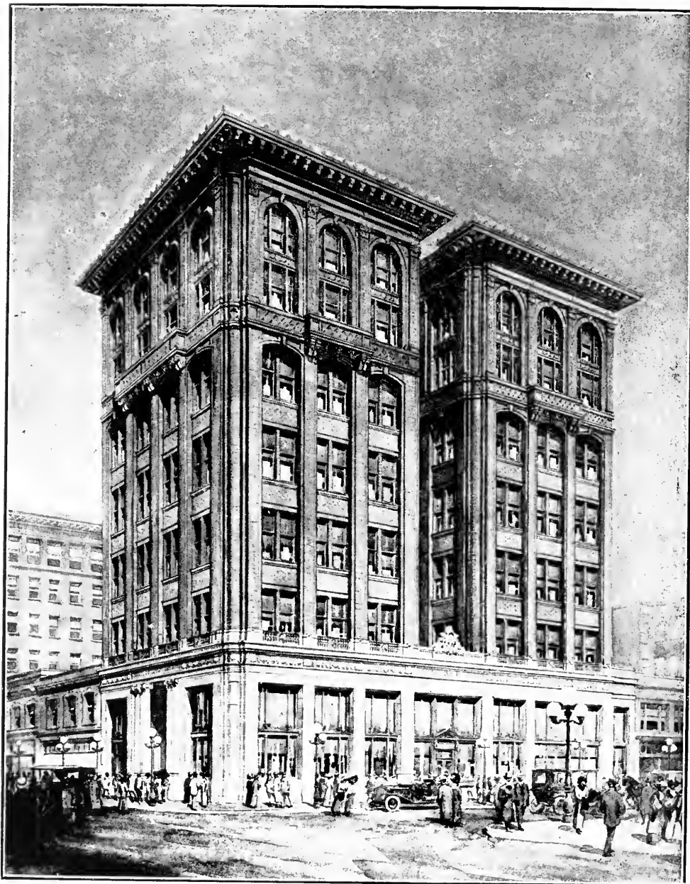
New Security Bank and Trust Company in course of construction at Eleventh and Broadway, Oakland
